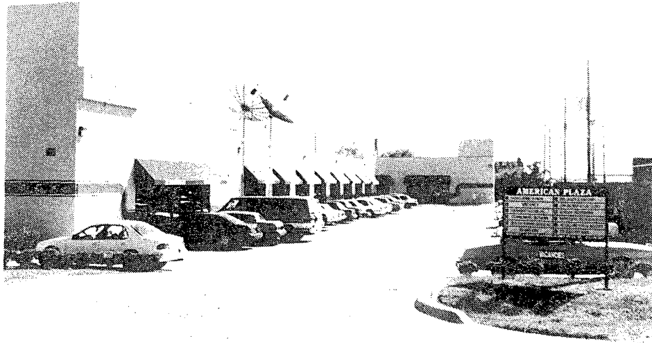
American Plaza. A project facilitated by BSEAT located at American Way and W. Camp Wisdom
