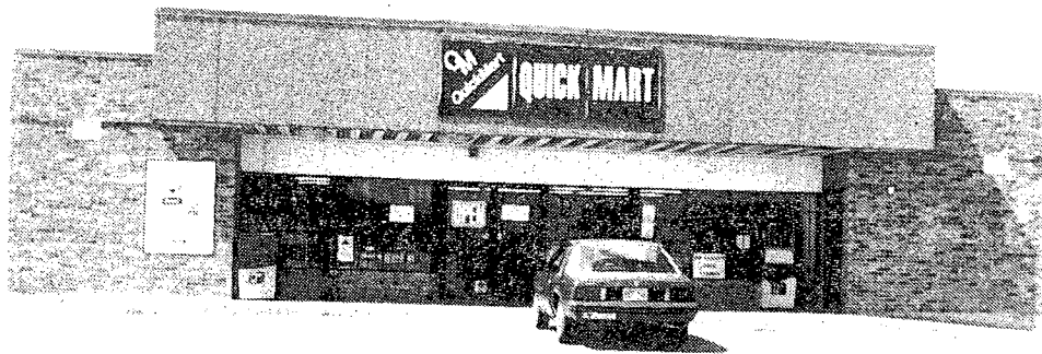
Former 7-11 Convenience Store. A project facilitated by BSEAT, located at S. Polk Street and Wheatland Road
